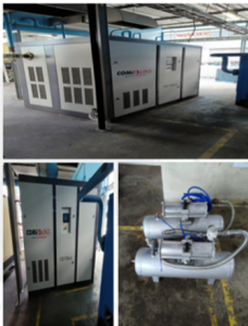
Project :Replace air compressor two stage
