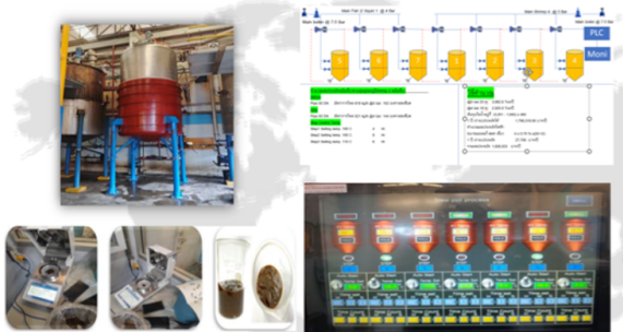
Project : Replace tank stew and Control valve
